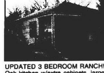
UPDATED 3 BEDROOM RANCH! Oak kitchen w/extra cabinets, large counters & nice table space. Reshingled roof, sun room/porch. Home Warranty. (17CEN) $111,900 734-455-5600
