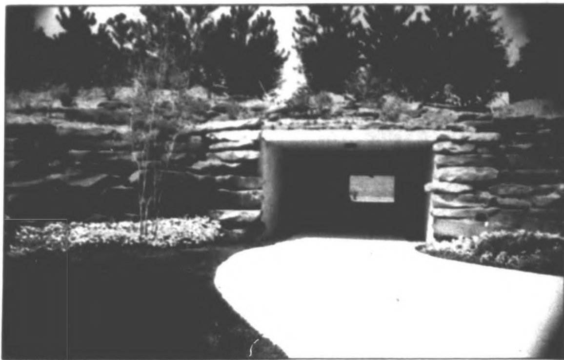
Instant access: A private tunnel beneath Orchard Lake Road provides property owners with safe, easy access from their lots to the water.
