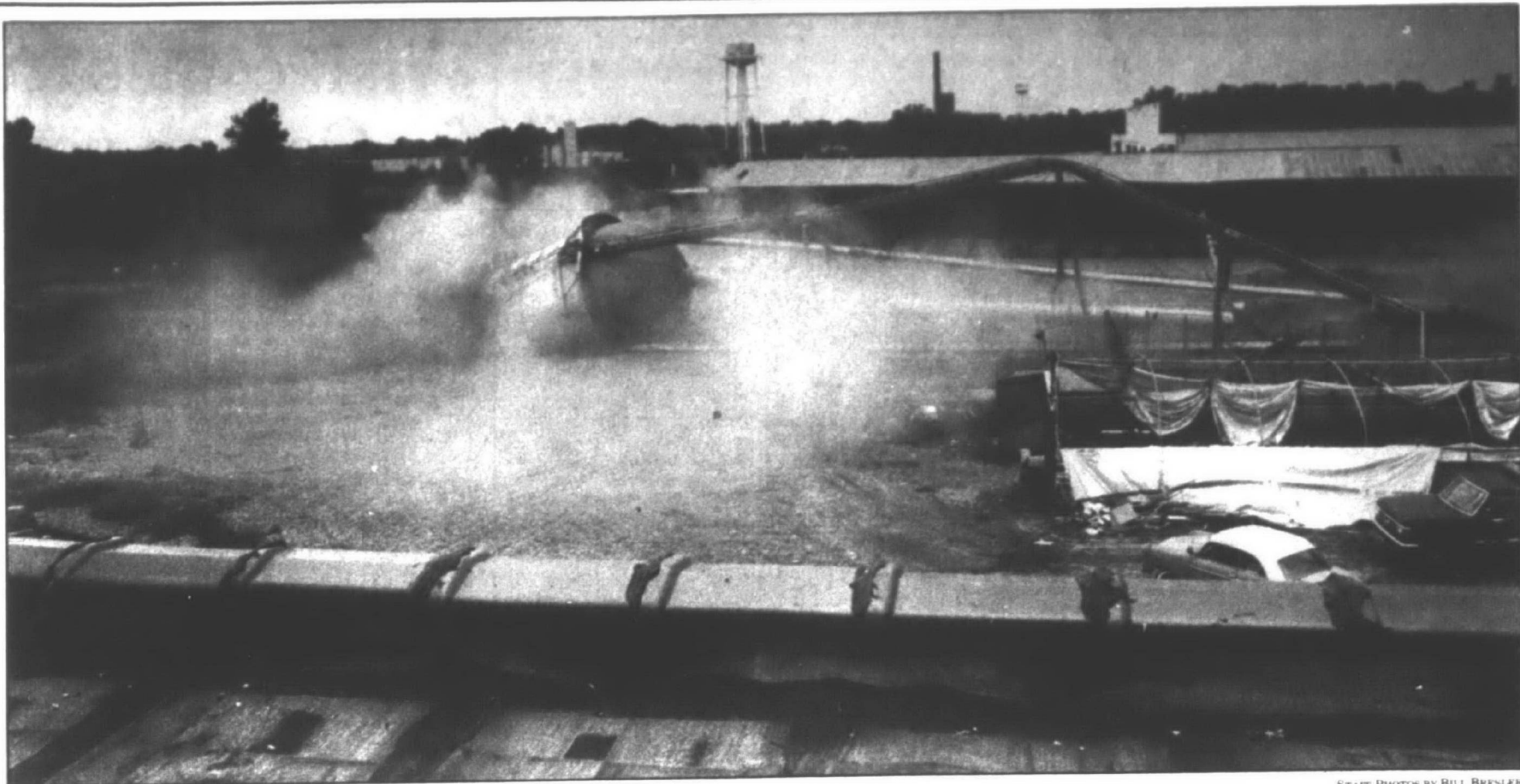
Raising dust: A crew from Federal Salvage turned the winch on a truck and down came the tower.
