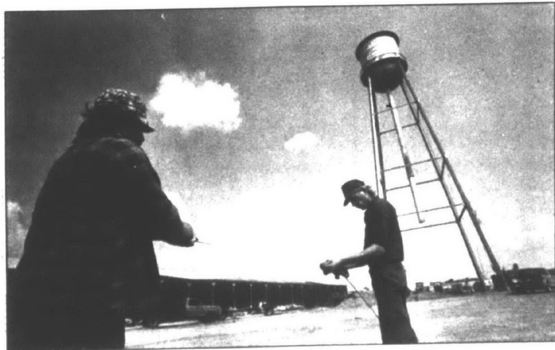
Measuring: Tracy Callis and Jeff Schultz measure the tower's height, 145 feet, to determine where it will fall.
