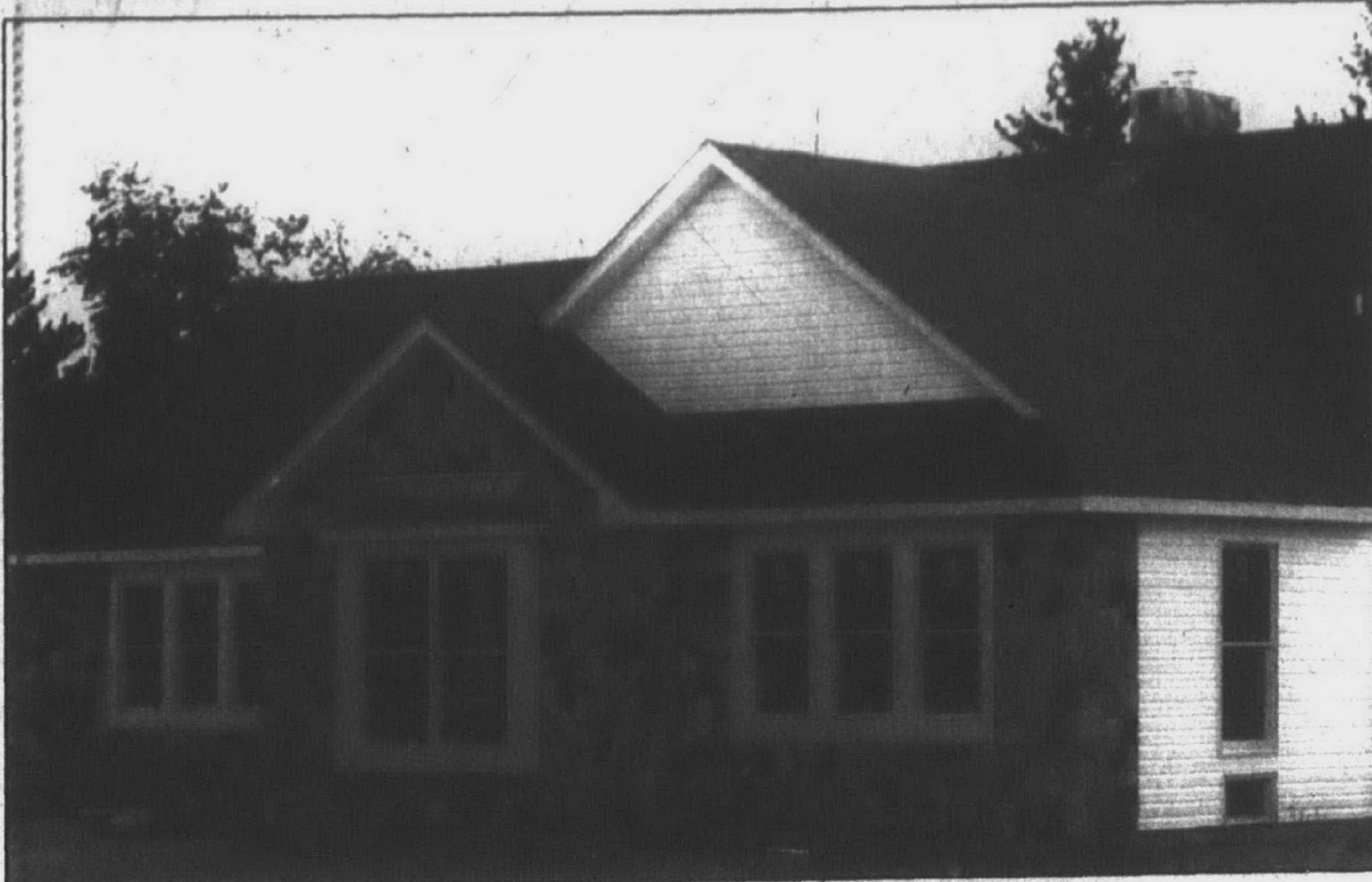
The front of this West Bloomfield home is a combination of Great Lakes Split Face manufactured stone and aluminum siding. Workers from Williams
