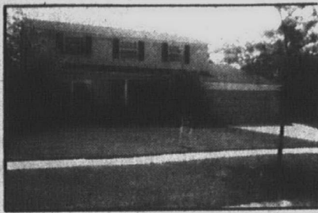
MAYFAIR VILLAGE. 4 bedroom, 2 1/2 bath Colonial, large family room, 1st floor laundry, master bedroom suite, all kitchen appliances, fenced yard, central air. (P84WES) $134,900 453-6800
