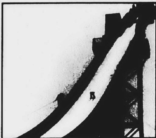
The copper Peak sky flying scaffold rises up 421 feet above the 364-foot summit of Chippewa Hill and has a vertical drop three times greater than that of Niagra Falls.
