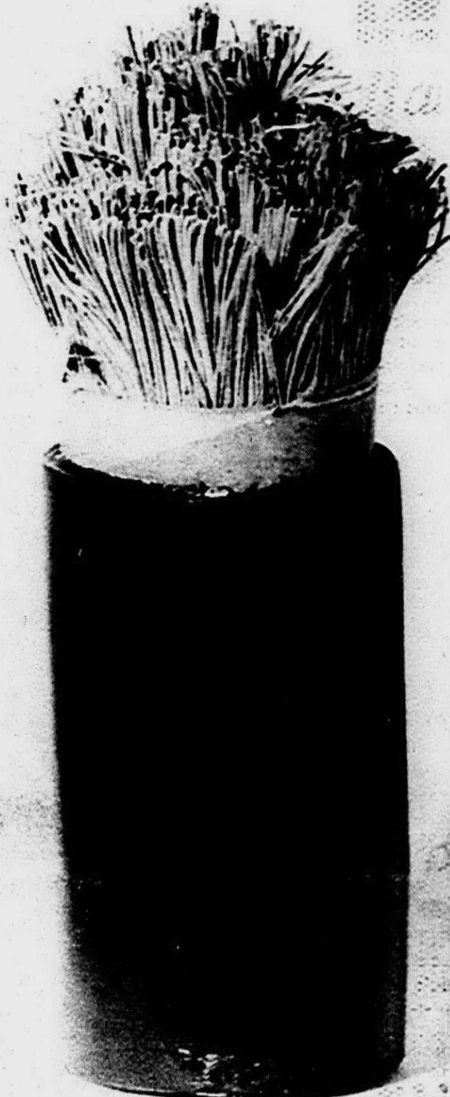
NEW SPRING PLANT? - APRIL FOOL — This is not a colorful spring plant, but a section of Bell Telephone cable showing 2,400 sets of wires that will permit 2,400 conversations passing through at the same time.
